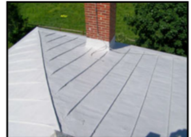
After Armor Roof
