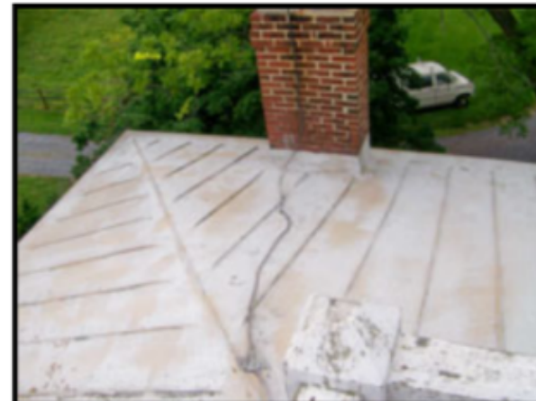
Before Armor Roof
