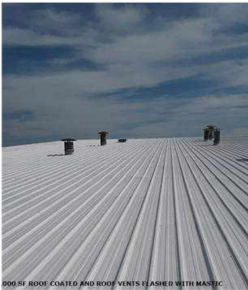
900 SF ROOF COATED AND ROOF VENTS FLASHED WITH MASTIC.
